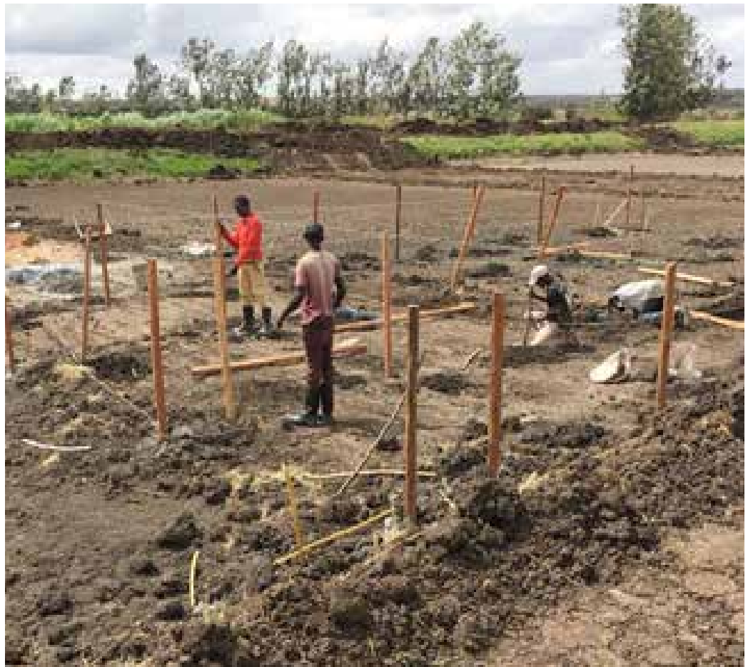
Construction of IPRS.
