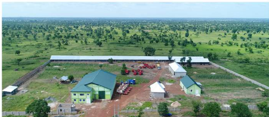
AERIAL VIEW OF CUDJOE ABIMASH FACILITY
