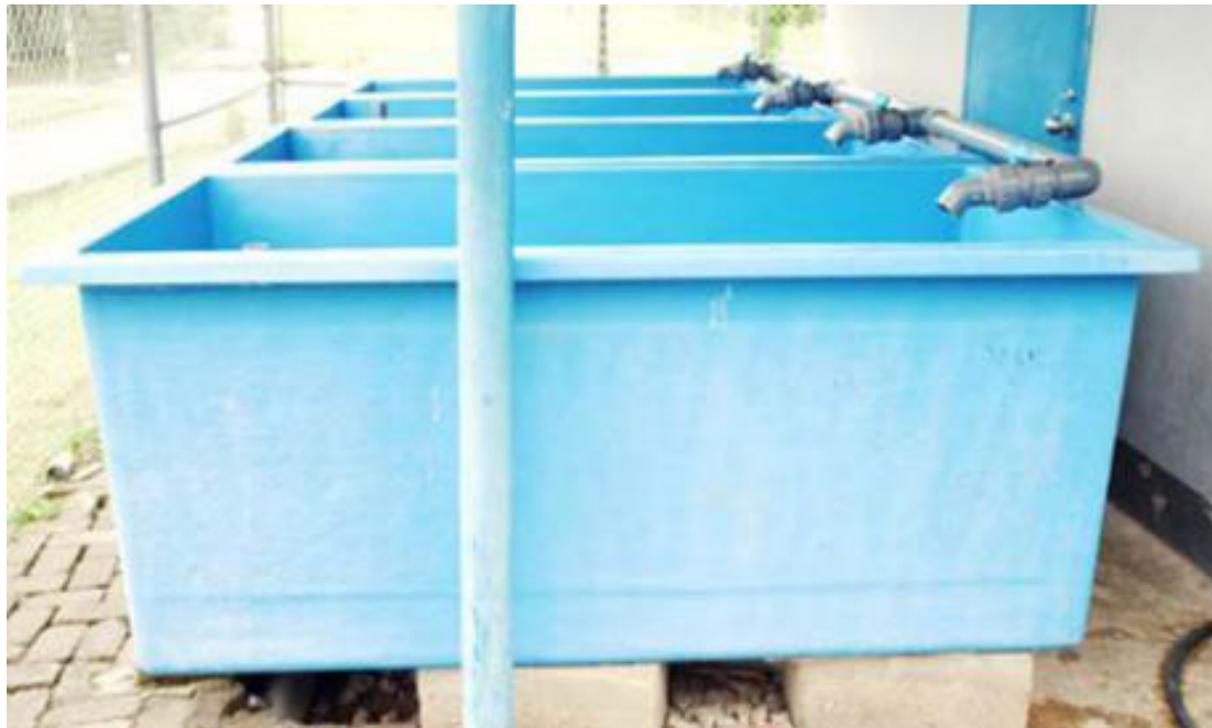
Flow-through tanks with single use of water
