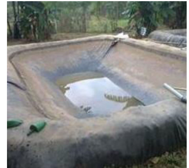
Excavated pond with liner
