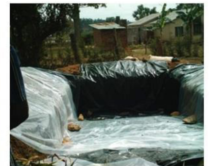
a) Digging a trench and lining it with plastic sheets
