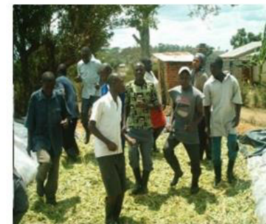
b) Filling the pit with material and compressing it for removing air
