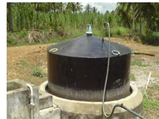
An aboveground biogas reactor; note the pipe used to bleed gasses at the top of the reaction vessel
