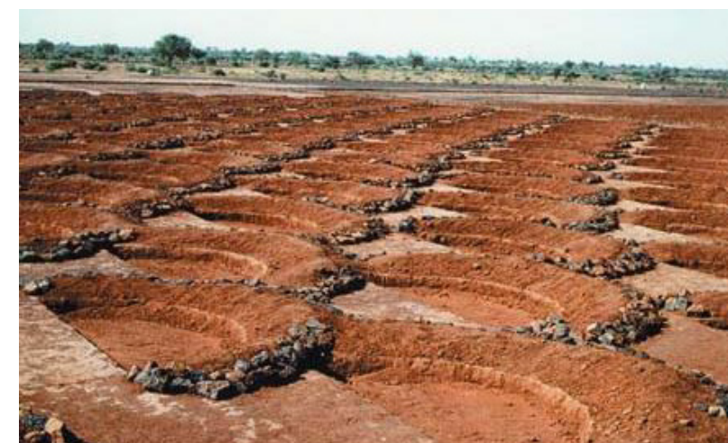
A network of half-moons reinforced with stones and intended to capture and direct limited rainfall
