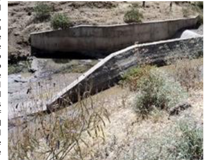
Diversion of a seasonal stream to feed spate irrigation
